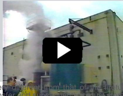
The operating principle of the Clayton Steam Generator is very different from that of the firetube boiler. A firetube boiler uses natural convection for heat transfer and subsequently it must store a large amount of energy in the form of high pressure hot water.
