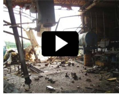
Overheating caused by low water is the most frequent cause of boiler explosions, or other damage. The most important job of the firetube boiler operator is to make sure the water level is correct at all times. In contrast a Clayton Steam Generator does not have a water level and it is not possible to have a steam explosion with the Clayton design.]
